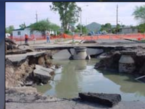
Emergency repairs to sinkhole, Tucson, 2002
