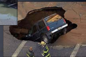
Sinkhole, Brooklyn, NY, 2006
